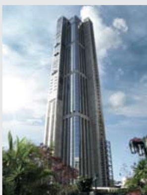
Venezuela Centro Simon Bolivar (56 Fl.) (Government Complex) • Caracas, Venezuela • Speed : 480m/min (2units), 420m/min (4units), 360m/min (2units) • Total : 15units
