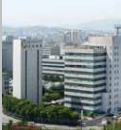
Icheon Head Office Factory 1, 2, and 3, R&D Center (size: 46,484m 2 )
