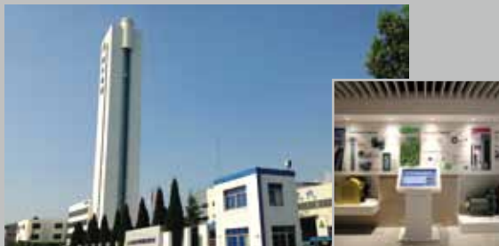
Shanghai Hyundai Elevator Co., Ltd. Manufactures elevators and escalators (size: 28,716m 2 ) Elevator test tower (height: 72m)
