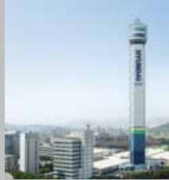
Hyundai Asan Tower A world-class elevator test tower (205m)
